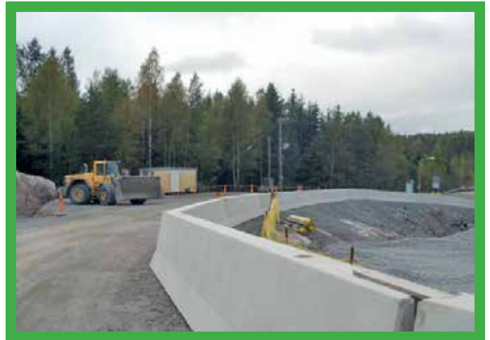
Edge Protection using precast structures.
